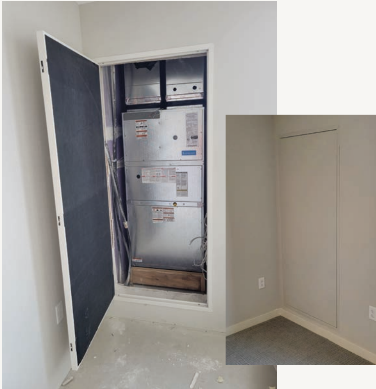
HVAC Access Door installation
