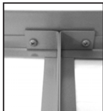
View of removable mullion from underside of access panel.
